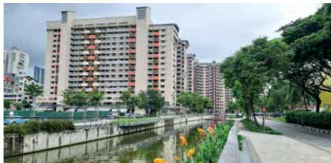
View toward Kelantan Court HDB Complex
