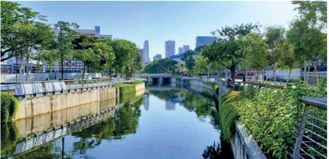
Rain gardens along the banks of Rochor Canal
