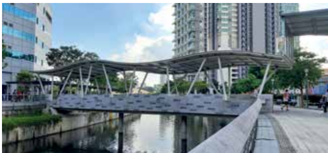
Wave Bridge, one of two pedestrian bridges that cross Rochor Canal
